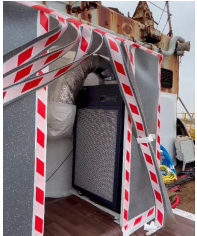
The dismantling and depollution process of ships emit potentially hazardous and harmful materials such as CMR (Carcinogenic, Mutagenic, Reprotoxic agents) and contribute to CO<sub>2</sub> emissions. In order to minimize the negative implications these materials can have on both working environment and the natural environment, Snadec contacted QleanAir France for a solution to the air quality challenges posed.
